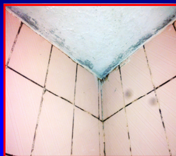
Black Funghi growing into Shower Tile Grouting
