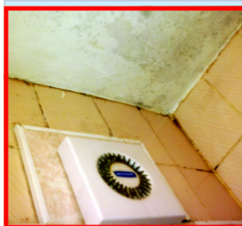
1. Surface Scum & Dirt Mould & funghi Growth
