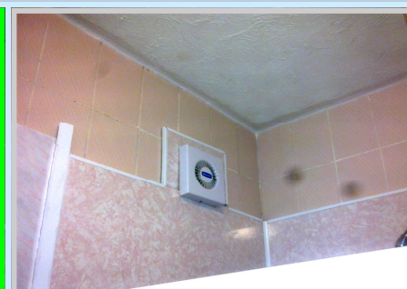
4. Stains removed, ESO Sealants applied, ALL grout waterproofed
