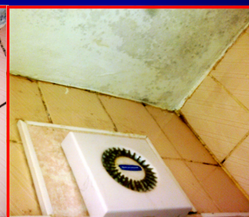
Black Funghi growing into Shower Tile Grouting
